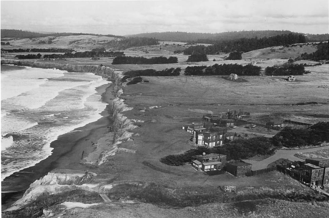
B5H Aerial view of Black Point Beach and the Esherick Hedgerow Houses. (c.1968) Photo by Lisa Trumpler
