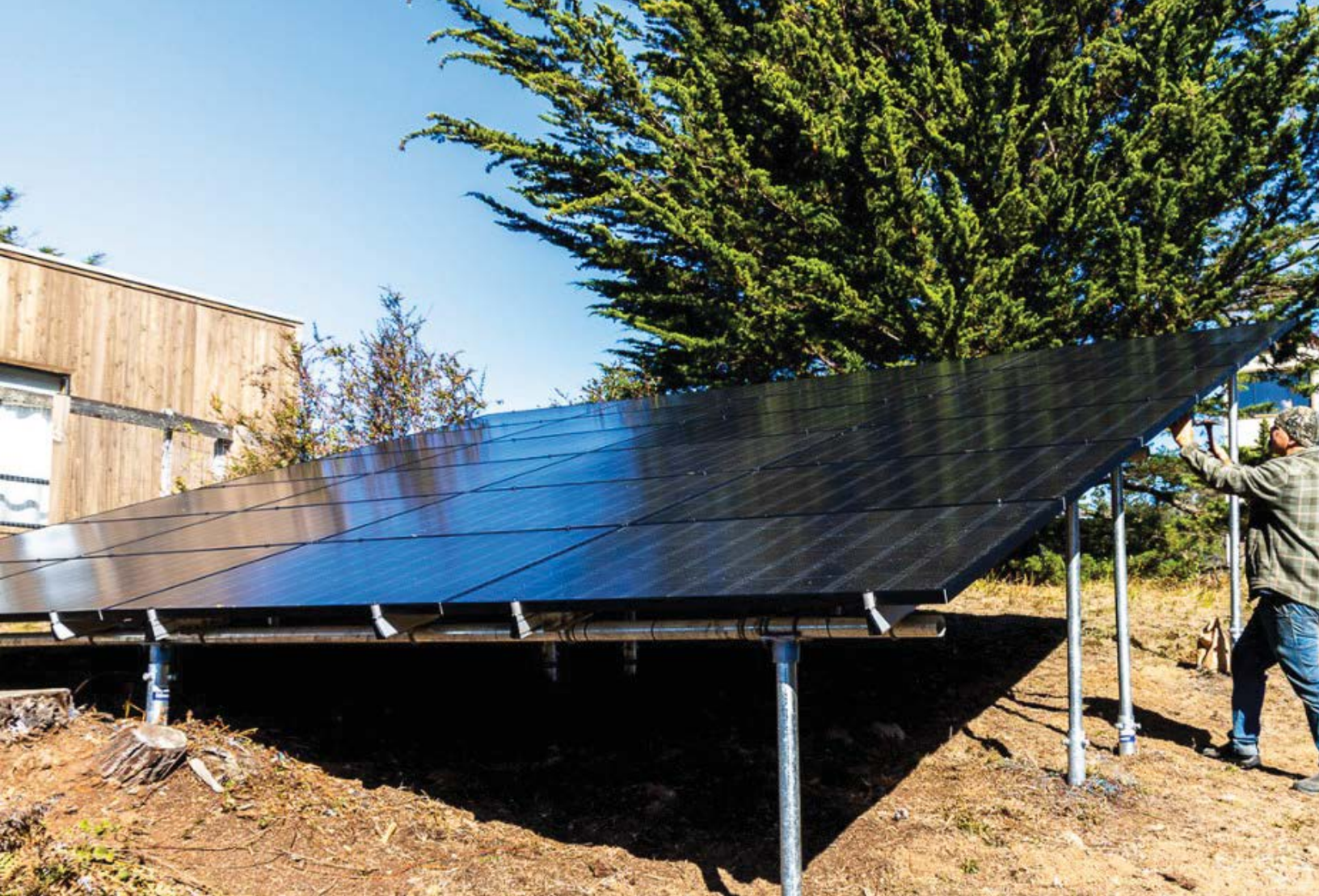
A ground-mounted PV system can capture the best exposure when a roof-line is shaded or not south-facing. Photo courtesy of M&D Electric.
