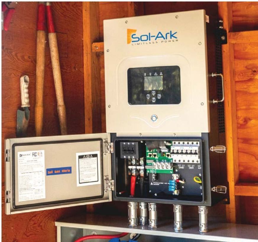
A solar inverter installed in a utility shed.
